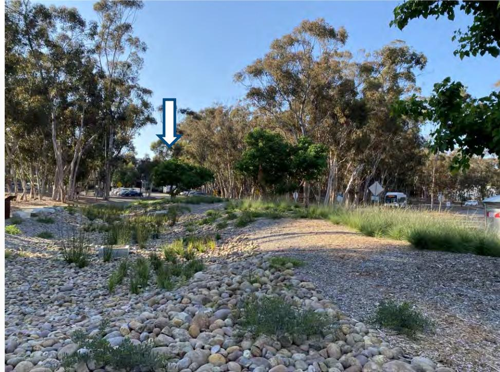
The campus replaced an asphalt road used for parking and a turf area with a stormwater treatment detention basin and drought-tolerant landscaping.
