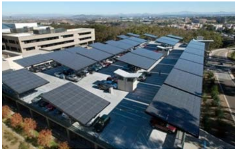
Solar Trees, Hopkins Parking Structure
